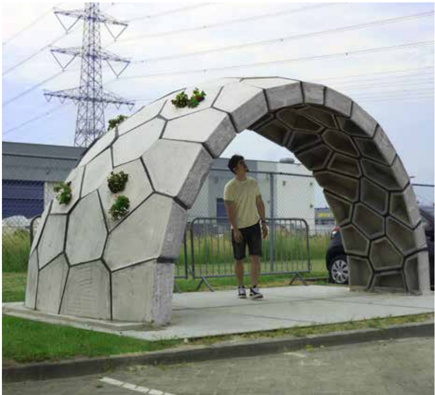
▲ The Green Dome consists of a housing that can only be made by the unique advantages of the 3D concrete printer.
