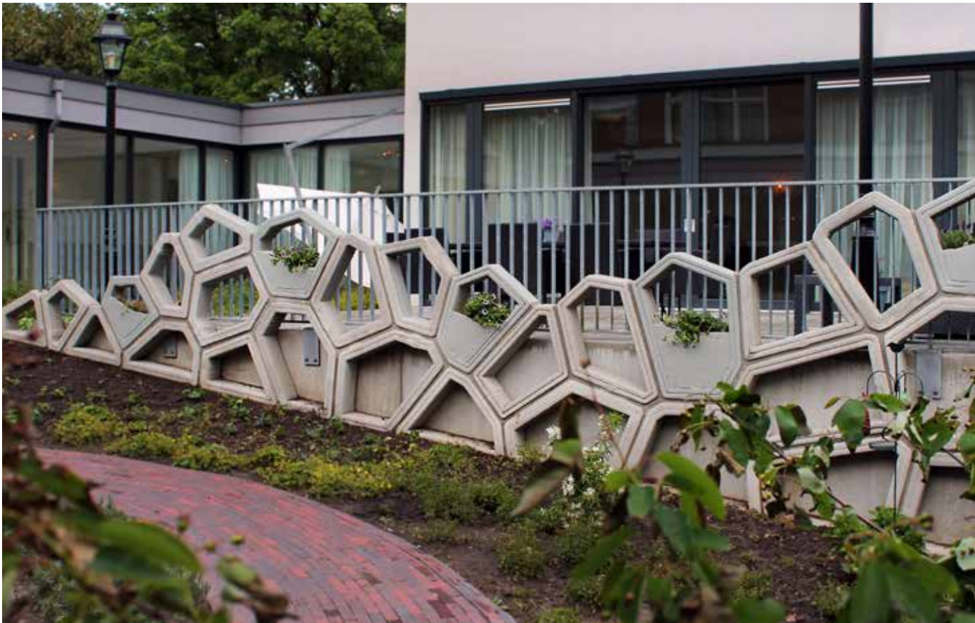
▲ The Saxion Betonprint Lab at Ariënsplein in Enschede has started using new software that makes it easier to make large-scale 3D concrete prints.
